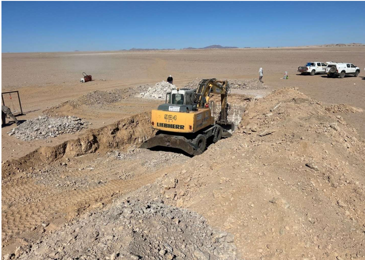
Figure 5 First Test Pit Excavated at Koppies
