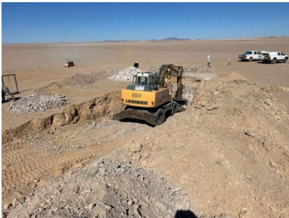
Figure 5 – Test Pit Excavation at Koppies Resource
